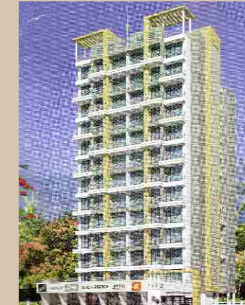
SILICON RESIDENCY ROADPALI, KHARGHAR
