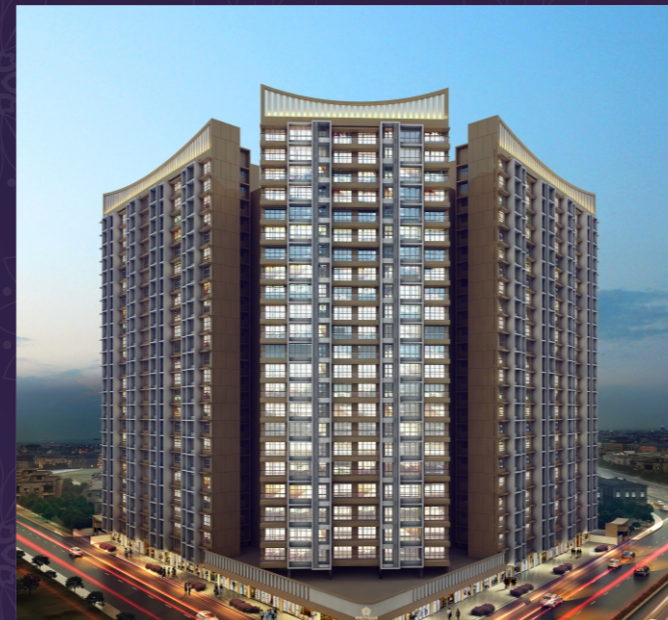
ANUTHAM - ONGOING MULUND (E)
