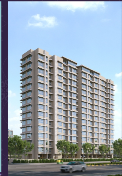
SILICON HOFE - ONGOING TILAK NAGAR
